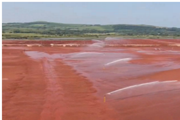
Figure 4. Automated sprinkler network operating on BRDA.
