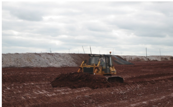
Figure 6. Bulldozing of carbonated bauxite residue.
